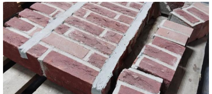
Figure 6. Cracking parallel to the groove due to the used hard epoxy glue
